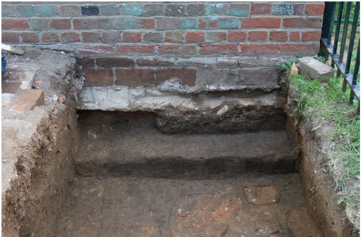
Figure 131. View of the Memorial Church foundations (facing west)
