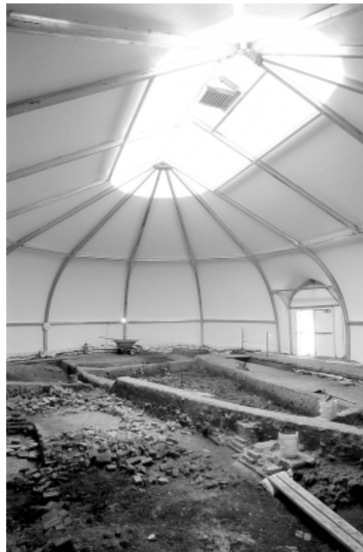
Figure 4. A view from the interior of the Sprung dome that protects Structure 163.
