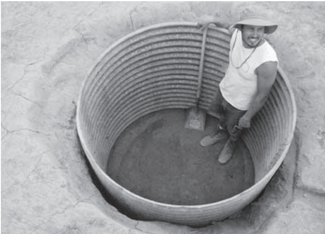
Figure 10. The well casing sits in partially excavated Well 1. The circular stain that marks the edges of the shaft and fill at this point in the excavation is smaller than the diameter of the casing.
