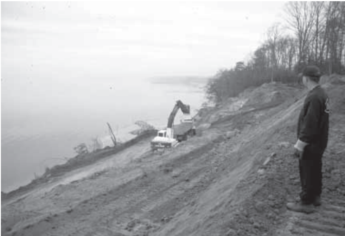
Figure 17. View of shoreline stabilization adjacent to Sandys Site.
